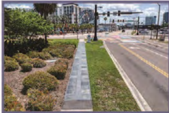
Solar Intersection Project Tampa, USA
